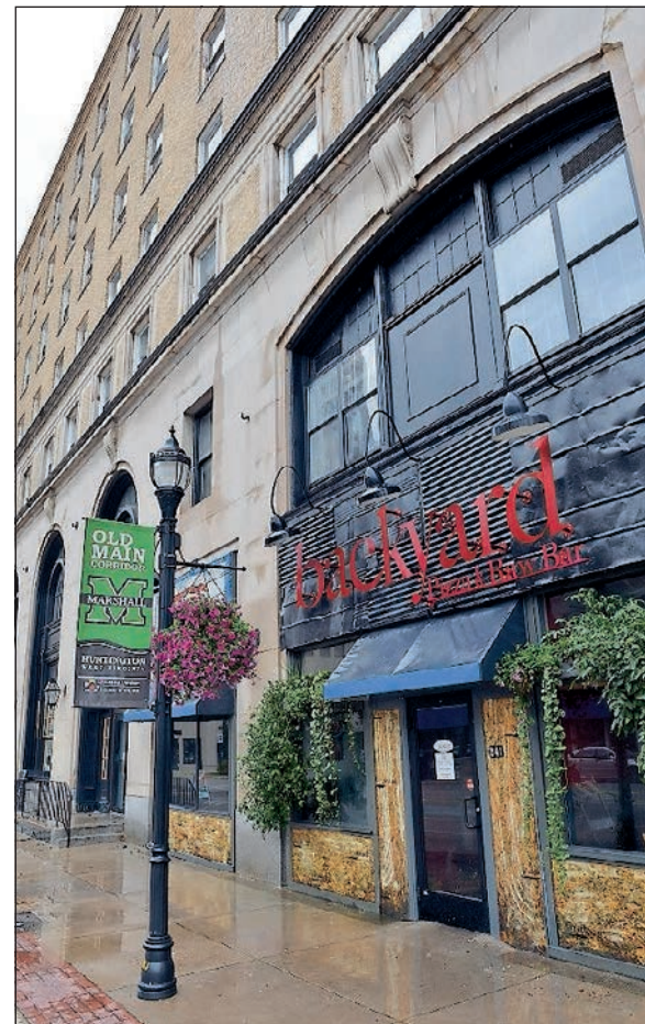
Water still drains out of the Backyard Pizza and Raw Bar.
